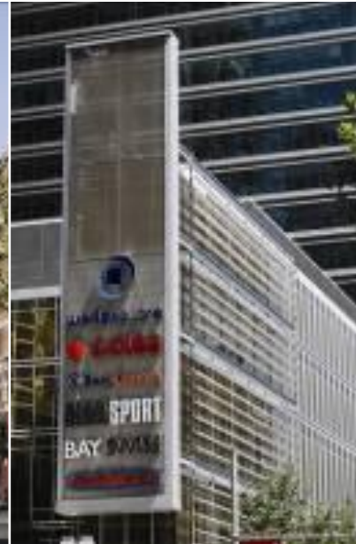
Sydney World Square Retail Complex and Public Car Park
